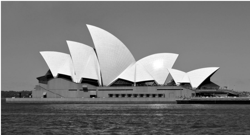
Figure 8 The foyers to the Drama Theatre and the Studio have undergone various changes over time. The conservation management plan identified these areas as being of some significance, with the various accretions being intrusive or of low significance. Utzon's proposal involves the creation of a sturdy loggia in similar materials, colours, and textures to the existing podium walls. The proposed loggia, shown on this computer-generated image, ensures that the planned openings in the podium walls are screened so as not to diminish the impression of the solid wall, but offers the opportunity to achieve Utzon's vision in which all the foyer spaces are connected visually to the harbour setting.
