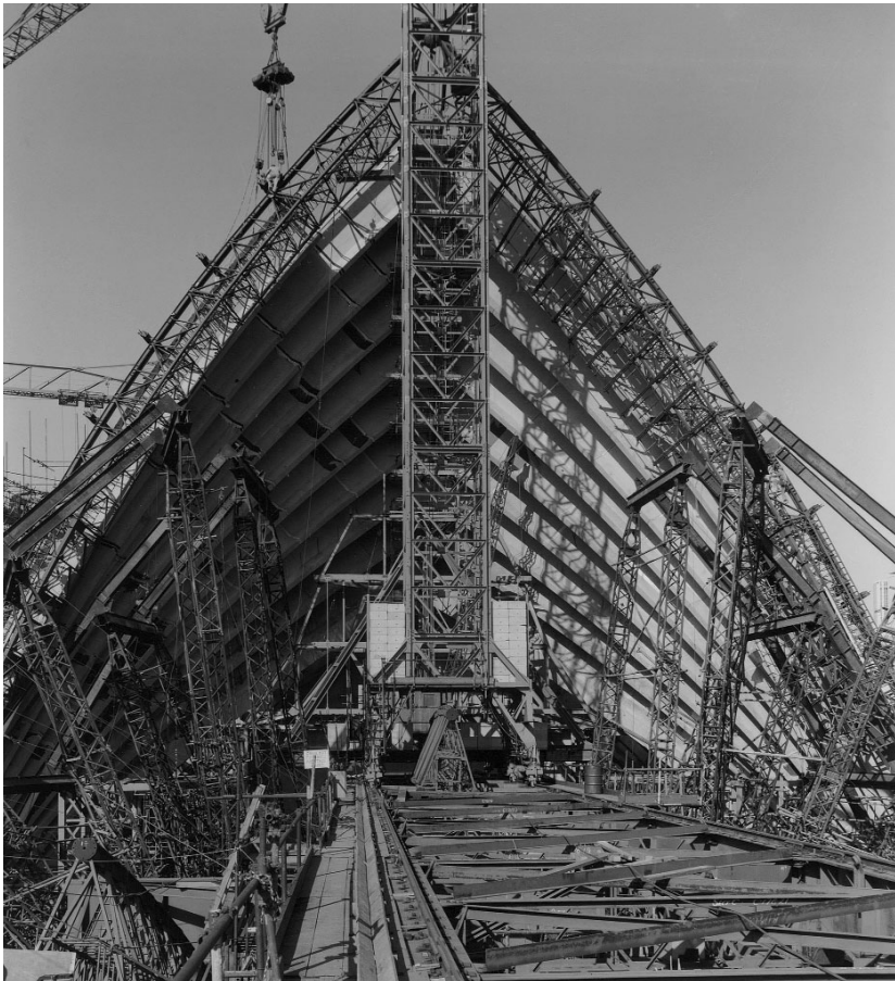
Figures 4 and 5 The brilliant solution to the construction of the roof shells was not identified until 1961, despite the fact that construction had commenced in 1959. Figure 5 illustrates the series of precast rib segments that rise from the podium to the ridge of the vault. The shells are clad in a pattern of matt and glazed tiles. (Courtesy State Library of NSW)
