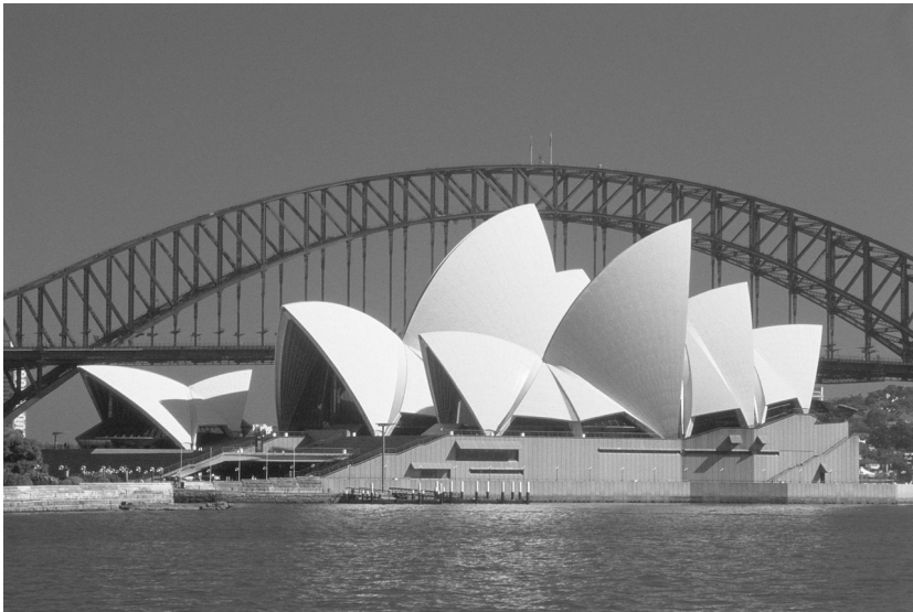
Figure 6 Stage I of the construction of Sydney Opera House, which commenced in 1959, included the building of the podium. Stage II involved the construction of the shells. Stage III comprised the remaining works to the building, including the interiors of the concert and opera halls, begun by Peter Hall following Utzon's departure in 1966 and completed in 1973. (Courtesy of Sydney Opera House)
